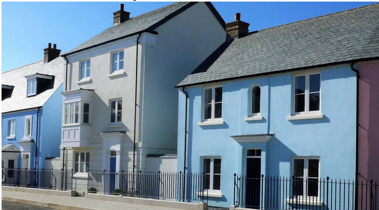
Figure 18 - New build in Nansledan
