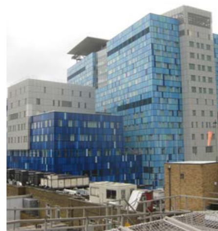
Royal London Hospital, Whitechapel. Before (top) and after (bottom) 3
