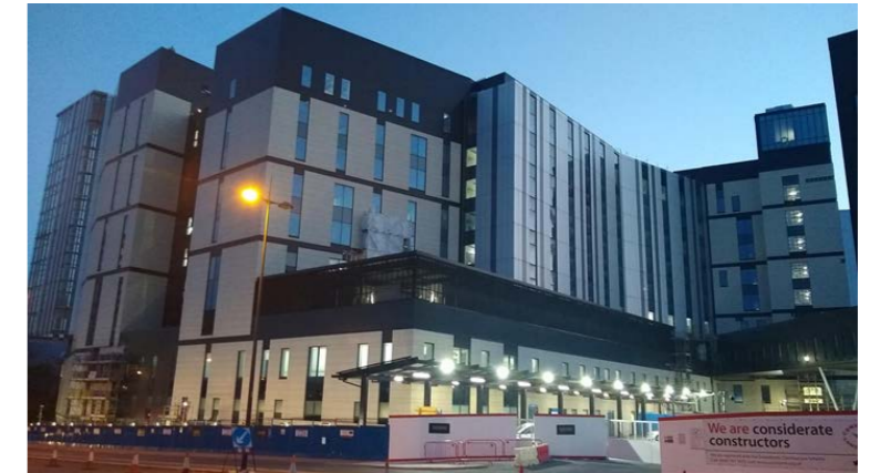
The new Royal Liverpool Hospital, Liverpool 52
