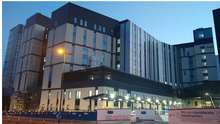
The new Royal Liverpool Hospital, Liverpool 52
