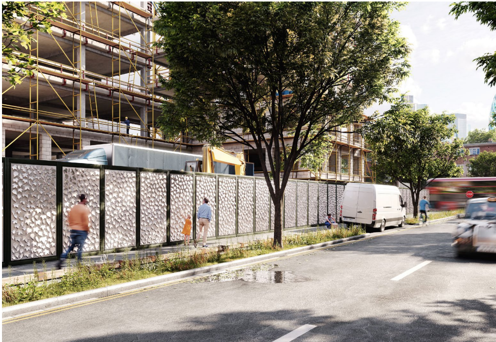
Author's design for a reusable panel for construction hoardings. The articulated design increases the available surface area for TiO 2 coatings
