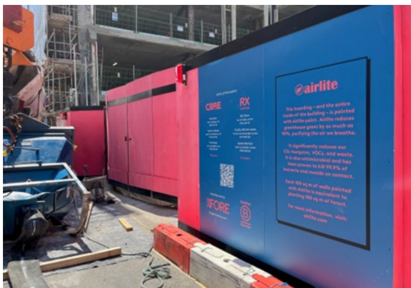
Pilot of TiO 2 coatings on construction hoardings, London. (Photo: Author's own)
