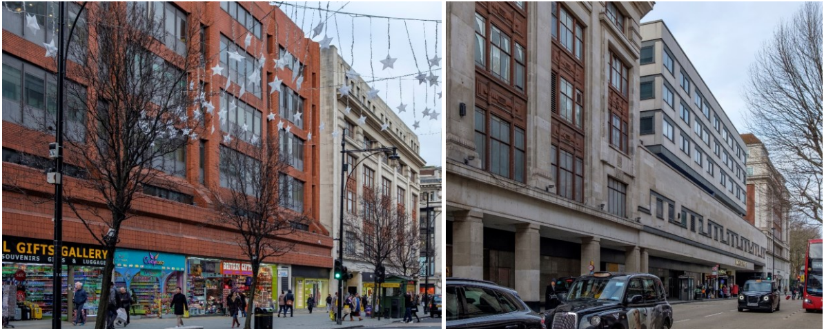
Post-war additions along Oxford Street (left) and Orchard Street (right)
