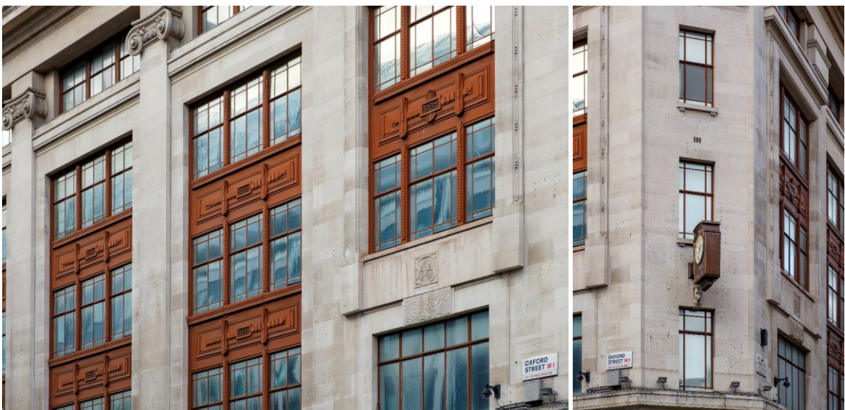
Façade details showing spandrel panels, pilasters and capitals
